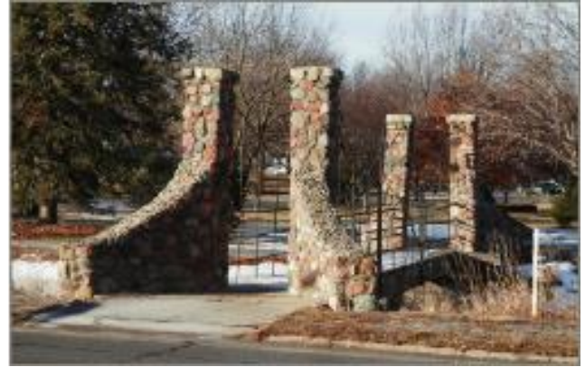
Figure 26. North Stone Footbridge (facing SW) Jan. 10, 2023
