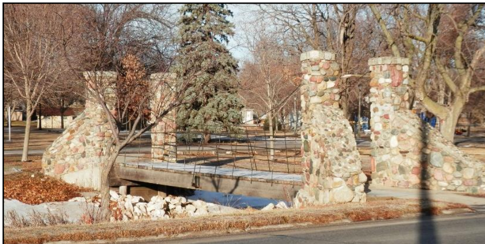
Figure 27. South Stone Footbridge (facing NW) Jan. 10, 2023
