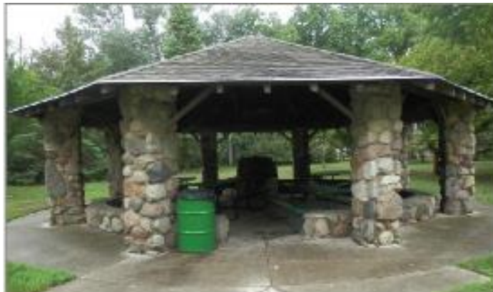
Figure 22. Open Shelter House (facing SW) June 6, 2023
