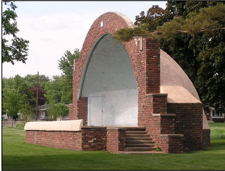
Figure 23. Band Shell (facing NE) July 1, 2017
