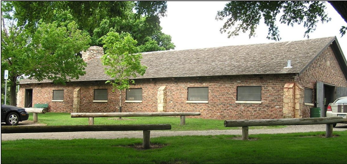
Photo 17. Enclosed Shelter House (facing NE) July 1, 2017
