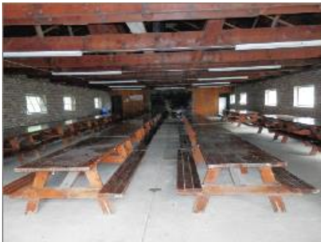
Figure 29. Enclosed Shelter House interior (facing N) June 6, 2023
