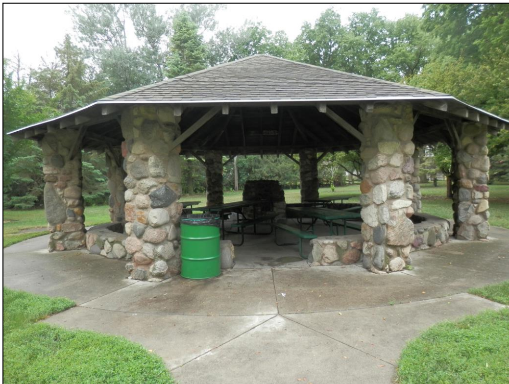
Photo 12. Open Shelter House (facing SW) June 6, 2023
