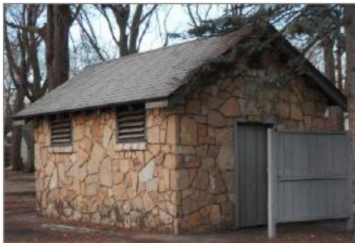
Figure 19. 1950 Restroom (facing SW) Jan. 10, 2023
