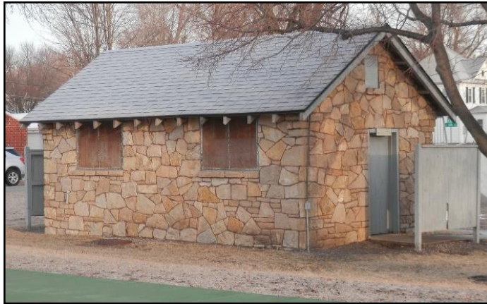
Figure 18. 1943 Restroom (facing NW) Jan. 10, 2023
