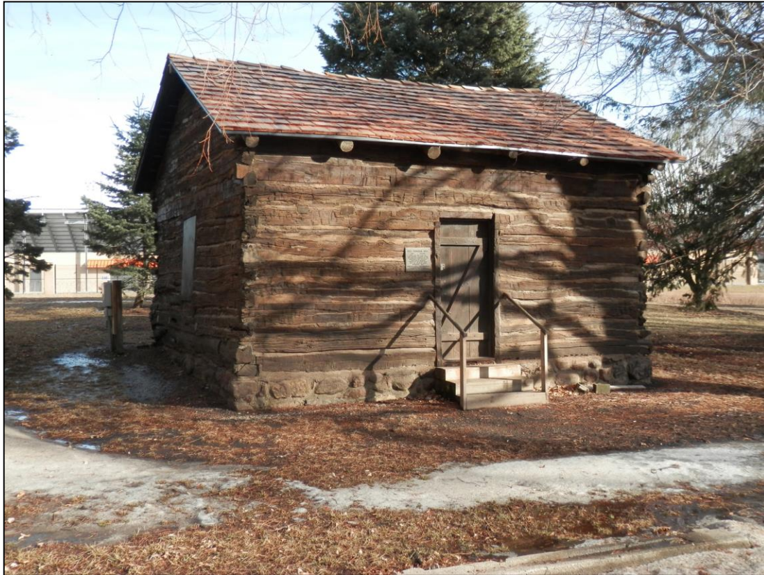
Photo 19. Trappers Cabin (facing SE) Jan. 10, 2023
