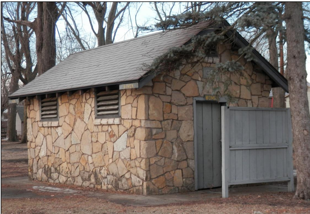
Photo 10. 1950 Restroom (facing SW) Jan. 10, 2023
