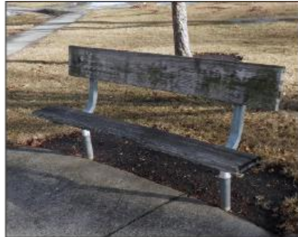
Figure 12. Wooden Bench (facing E) Jan. 10, 2023
